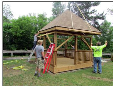
Pre-constructed gazebo is lifted into position
