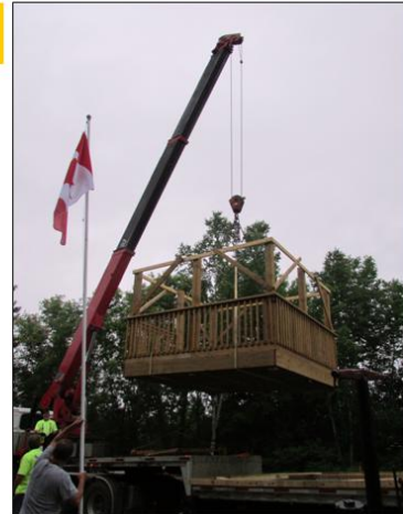
Pre-constructed gazebo is lifted into position
